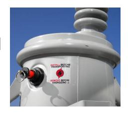
Pressure relief valve...pull the ring to operate manually
